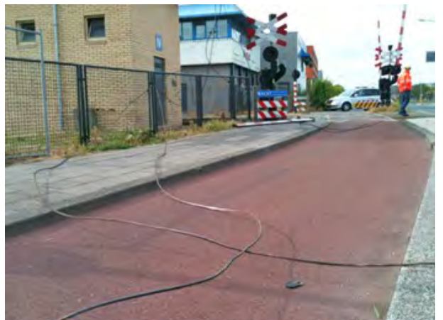
The remains of the electrical cables of a railroad after collision with an overheight trailer
