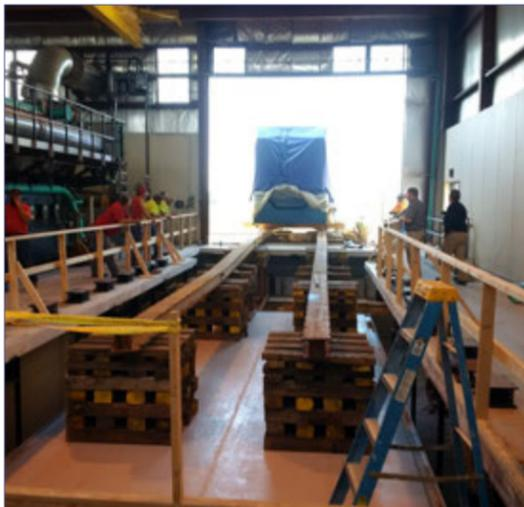
breakbulk cargo delivered the city's second generator set in an effort to expand its power generation capability.
