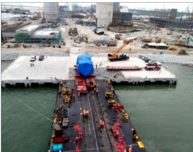
timely Ro-Ro operation at Jimah site jetty given the limited tide due to the height of the jetty.
