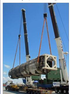
industrial equipment for a fructose plant, consisting of 12 units, each weighing between 25 and 100 tons, with a total weight of 701 tons. The largest unit was 28 meters long.
