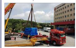
Freight Link Express' bonded ware-house. The freight forwarder used a 150-ton crane to unstuff the equipment from the flat rack container onto a low loader, for trucking to the Malaysia factory. www.gpln.net
