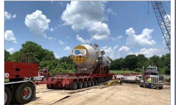
safe bayou offloading facility adjacent to the swollen Mississippi river. Continual heavy rains in the Midwest and southern states has caused an alarming rise in the water level of the river and treacherous currents threatened the successful delivery of the reactor for parties involved.
