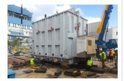
n the 27th January 2020, GPLN member Egyptian Global Logistics (EGL), a subsidiary of KADMAR GROUP, completed jacking/skidding of 3 transformers (116 tons each) for SIEMENS in Abu Qir Substations.
