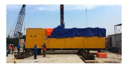
ing to safety conditions. The crane 360T lifted up all part of enclosure and engines at the top of the building. After all parts of engines were assembled, the unit was rotating 90 degrees, using jacking & rolling equipment. A prudent survey, operating plan analysis, routes and type of transportation were the key factors of a success
