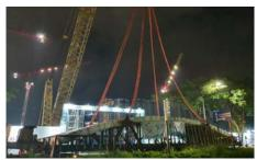
PLN member Super Cargo Transport from Vietnam is glad to announce that a big acrylic panel was safely delivered from discharging port to jobsite in May 2021. They came up with a solution for direct receipt under hook at berth, temporary storage at storage yard and safe delivery to the jobsite. Dimension and weight: (L)18,85m x (W)6,85m x (H) 2,49m and 65.5 tons.
