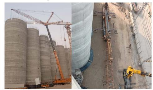
cent Syndicate" have provided Erection & Placement Services at Volka Food Multan, Punjab. Our work–scope included the erection of Silo–Tops and placement of the aforesaid tops onto multiple Silos at Volka Food Factory Multan, by using
