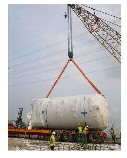
the bank of Shitalakshiya river, nearby the project site, to discharge cargoes by using 150ton capacity lattice-boom, crawler crane, which was set on that barge.
