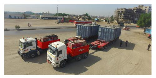
PLN member M/s M. Amin M. Qaseem (Pvt) Ltd., one of the leading and pioneer one—stop project logistics solution providers in Pakistan, has recently handled and delivered the shipment of 2\*220 KV Transformer main bodies (weighing 146 tons each) from Karachi Port to 220 KV Grid Station
