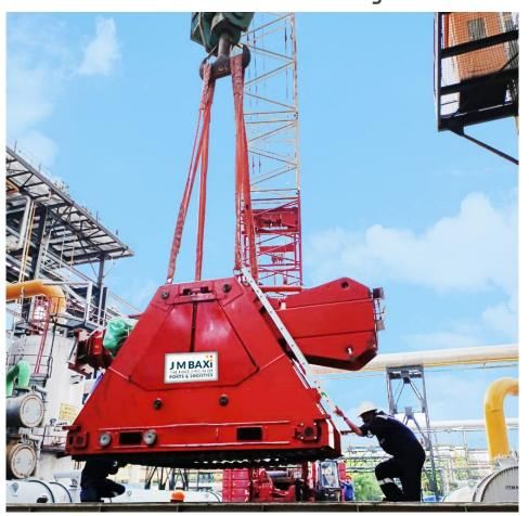
ndertaking a truly intricate endeavor at GAIL Vijaipur, GPLN member J M Baxi Heavy from India embraced a complex task that involved replacing three imposing condensers, each measuring 14 meters in length and 1.9 meters in diameter with a total weight of 101 metric tons.
