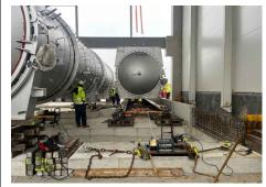
For the internal movement at beneficiary's premises, we have used a tailor-made system engineered, built and operated by our crew. We designed and constructed robust trolleys, each capable of supporting 45 tons, and mounted them on rails.
