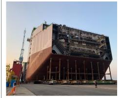
CTC Transportation company from Korea sourced Cometto self-propelled modular trailers (SPMT's) to load out FPSO components with a combined weight of 63,781 tons in South Korea.
