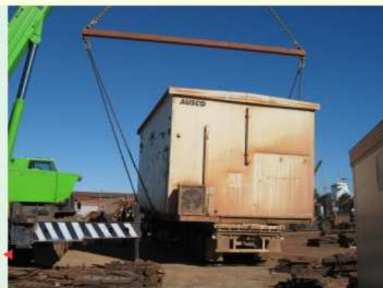
Electrical Control Building being loaded at Port Hedland Laydown
