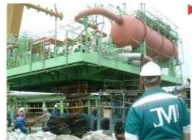
▶ EPSO Topside Process Module; 35 x 28 x 10 mtr, 850 MT
